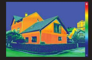
Without continuous insulation, heat loss through framing (thermal bridging) is significant.
